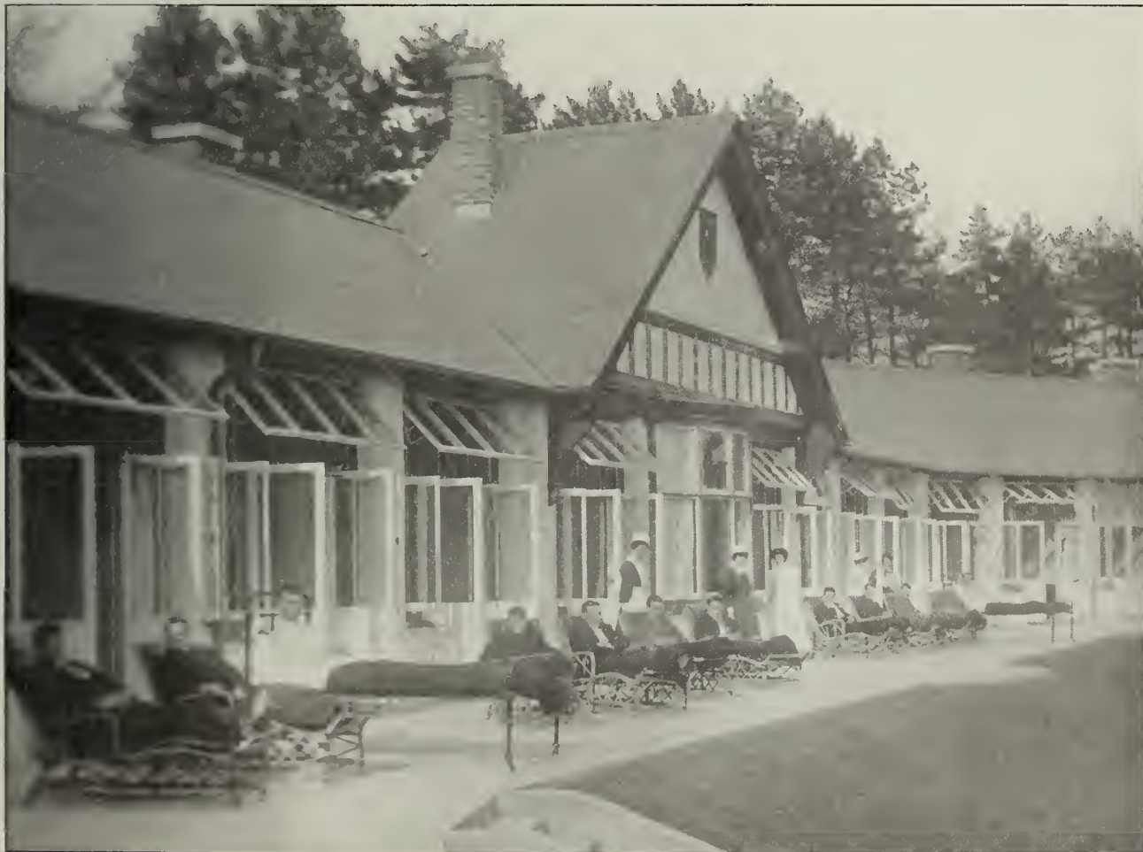
1.—Section of open-air Sanatorium at Salterley Grange opened in 1909. Here cases of tuberculosis are treated all the year round in the open air, the rooms being for the most part needed during wet or doubtful weather only. Colds or ill effects of the open air are unknown under these conditions.
